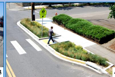
Image 3 shows an inadequate pedestrian bump out on Main Street in Downtown Mount Clemens. Bump outs increase safety by improving pedestrian and vehicle visibility to those who are using the crosswalk. In addition, pedestrian bump outs increase pedestrian comfort by decreasing crossing distance. Image 4 provides an example of a bump out in Seattle, WA that is well defined from the roadway. Raised curbs and landscaping prevent vehicles from entering pedestrian space.
